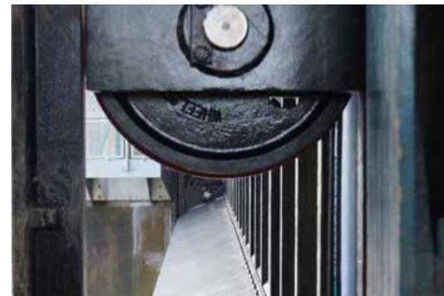
The project included the replacement of the steel ropes and the gate runners which guide the sluice gate into position during normal operation. It also involved a specialist dive team to install two limpet cofferdams which allowed the engineers to remove and replace the gate running tracks under dry conditions.
